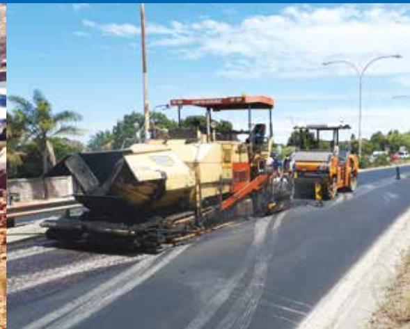
*Paving of bitumen rubber asphalt base (28mm Colto BTB with AR-1) to fast and slow lanes of Durbanville Avenue.*
