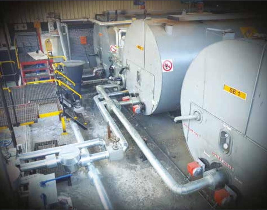
*The modified plant incorporating a high shear mill to produce PMB in Alrode.*
