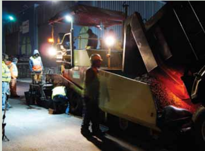
Paving at OR Tambo International Airport.
