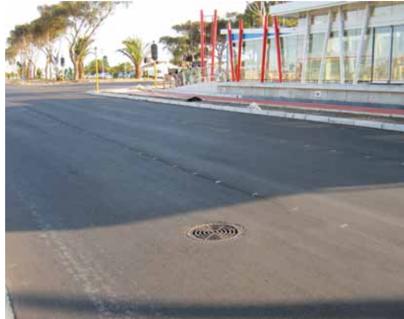
Bus on/off point in Tableview Road.
