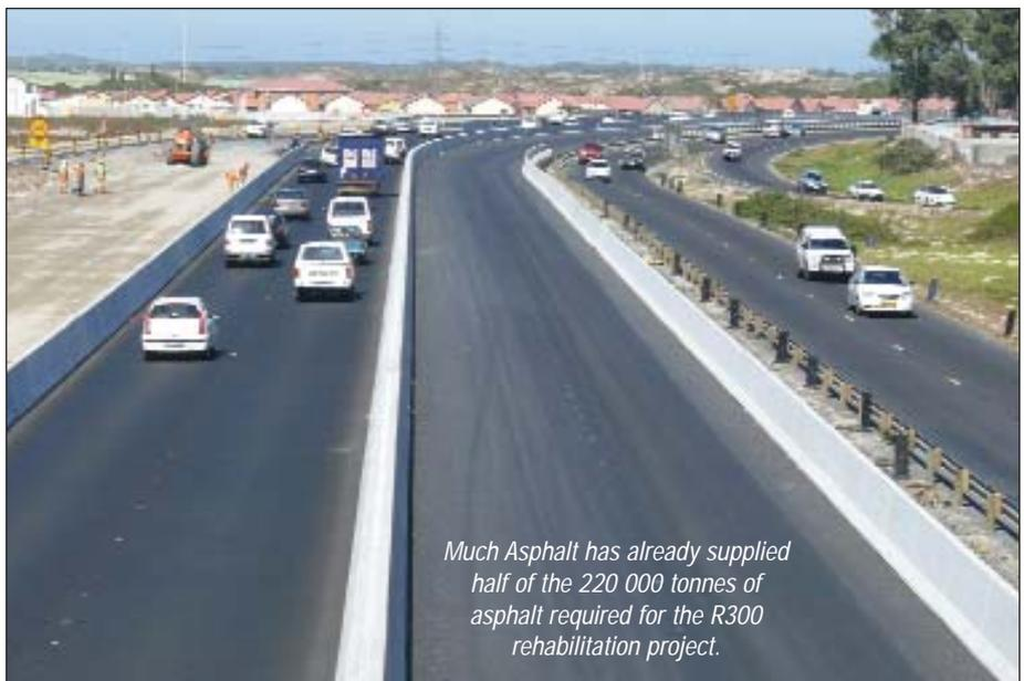
*Much Asphalt has already supplied half of the 220 000 tonnes of asphalt required for the R300 rehabilitation project.*
