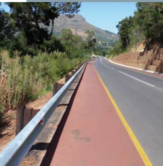
Red asphalt promotes safety in Pniel.
