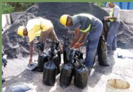
Bagging of cold mix from stockpile.
