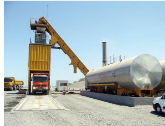
Ermont drum plant on the Grand Bois bypass project.
