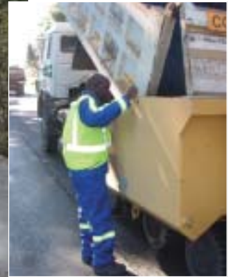
Johnson Burwana of Much Asphalt tests the asphalt temperature.
