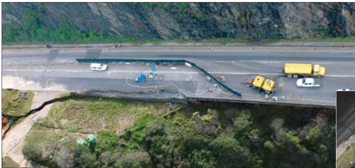
This aerial view shows the magnitude of flood damage to the Kaaimans River Pass on the N2 between George and Wilderness.
